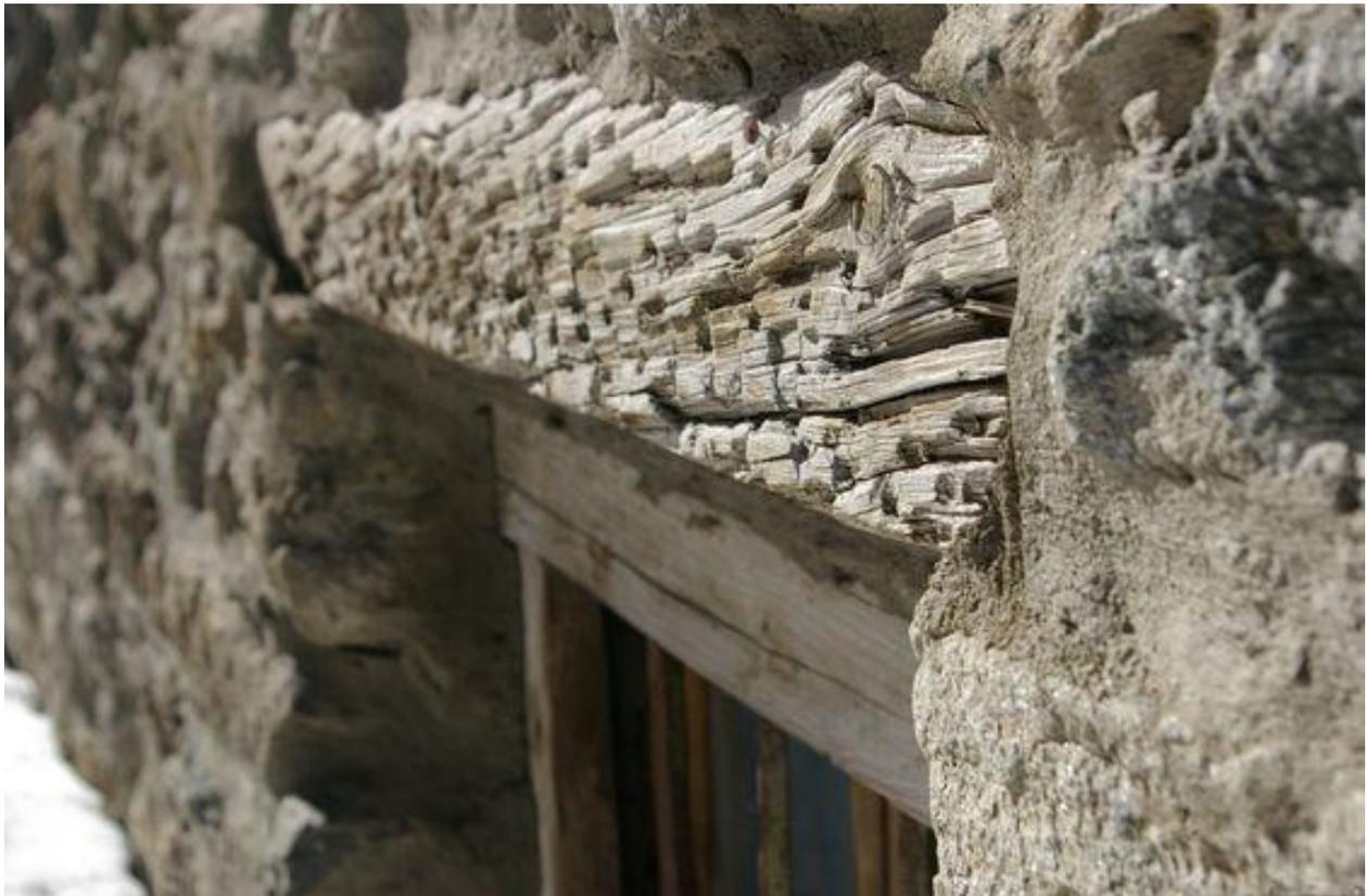
*Figure 1: The surface of the support beam is roughened in the interest of providing ideal surface to plaster (Pinterest 2020a)*
