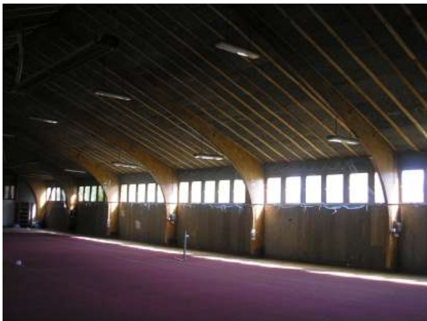
Figure 1: Glued-laminated structure made of poplar
